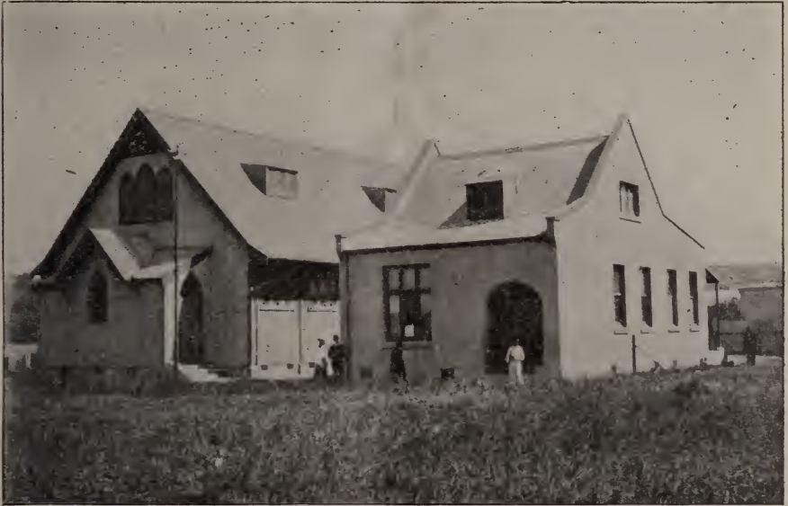
CHURCH AND DISPENSARY AT DURBAN
